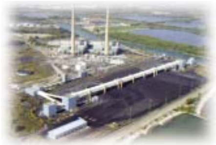
Coal blending is an effective means of achieving greater operational flexibility for the existing coal fleet. Detroit Edison's 3,000 MW Monroe plant blends three coal types in an almost infinite number of recipes to fit specific market conditions. Photo courtesy of Detroit Edison.
